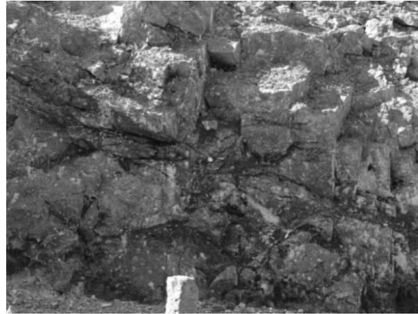
Figure 2. Image showing blocky nature of the granite rock mass at the Tremough Campus road cutting.
