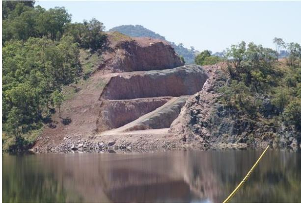
SunWater engaged a CAE Mining consultant to undertake both geological and structural mapping and analysis of a spillway wall using Sirovision technology. The mapping was required for a stability analysis of the natural outcrop at the dam site. Sirovision technology provided a fast, safe and remote mapping capability for mapping the structure.
