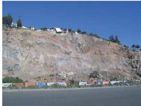
Figure 4. Overview of the Peacock's Gallop field site. Note the paleochannel in the central upper part of the cliff and the use of shipping containers as rockfall barrier.
